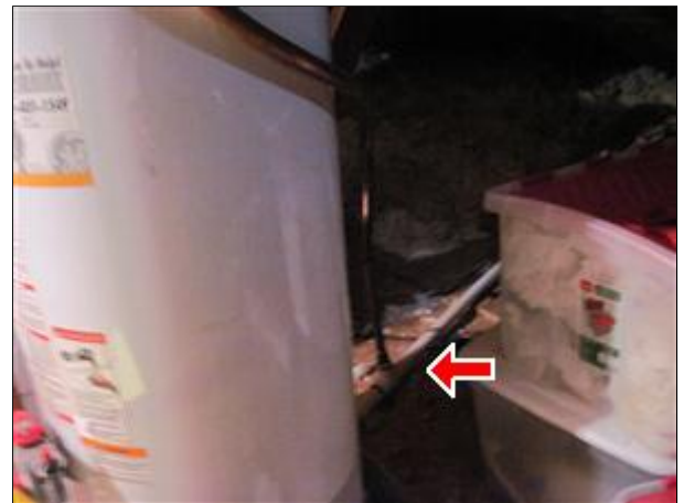
C. Picture 6 TPR tied to pan drain
