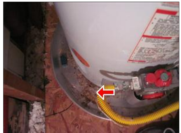
C. Picture 8 Debris in pan
